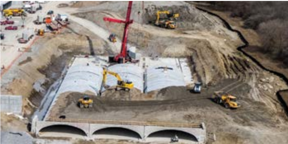
Overhead view of installed precast stormwater structure
